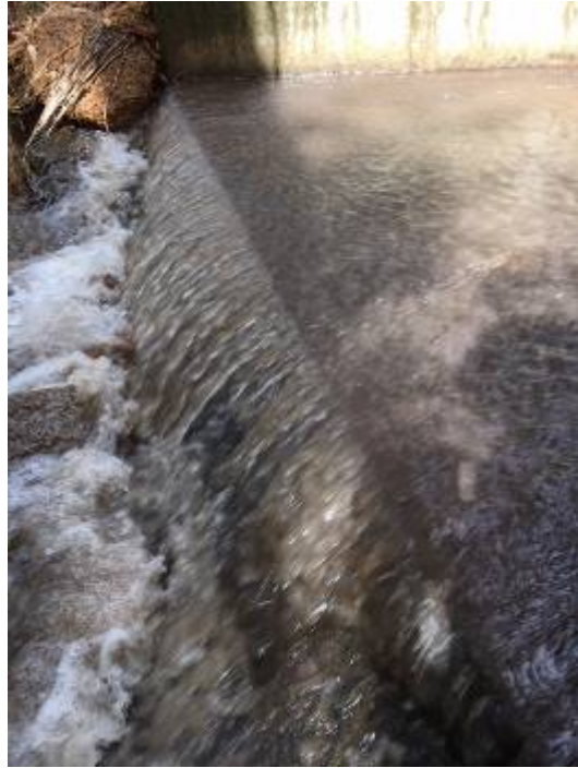
Over the current spillway
